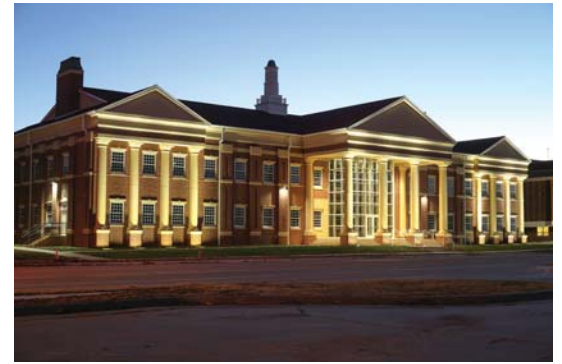
Jane E. and Nick K. Stavros Hall is the home to the OBU College of Nursing. This 32,000-square-foot facility is designed to provide cutting-edge nursing education for both undergraduate and graduate-level students.
